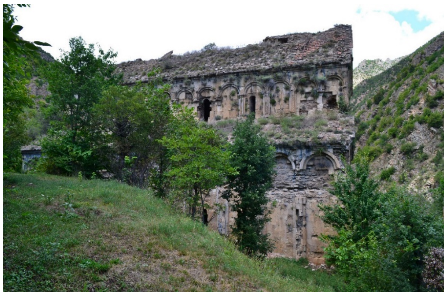
Fig. 3. General view from the north (Canöz's Archive).
